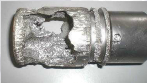
Figure 4. Wrong plug material selection.
